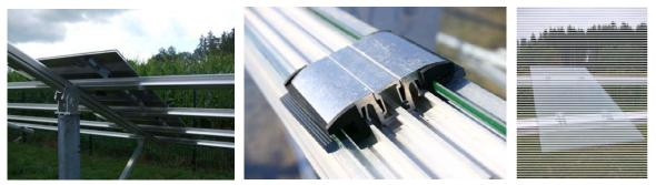
Fig. 1 General fixation concepts (backrail / clamps / spot fastener)
